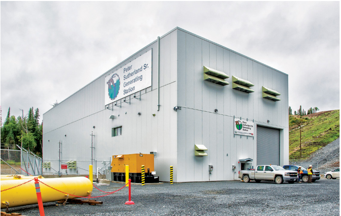
Peter Sutherland Sr. Generating Station
