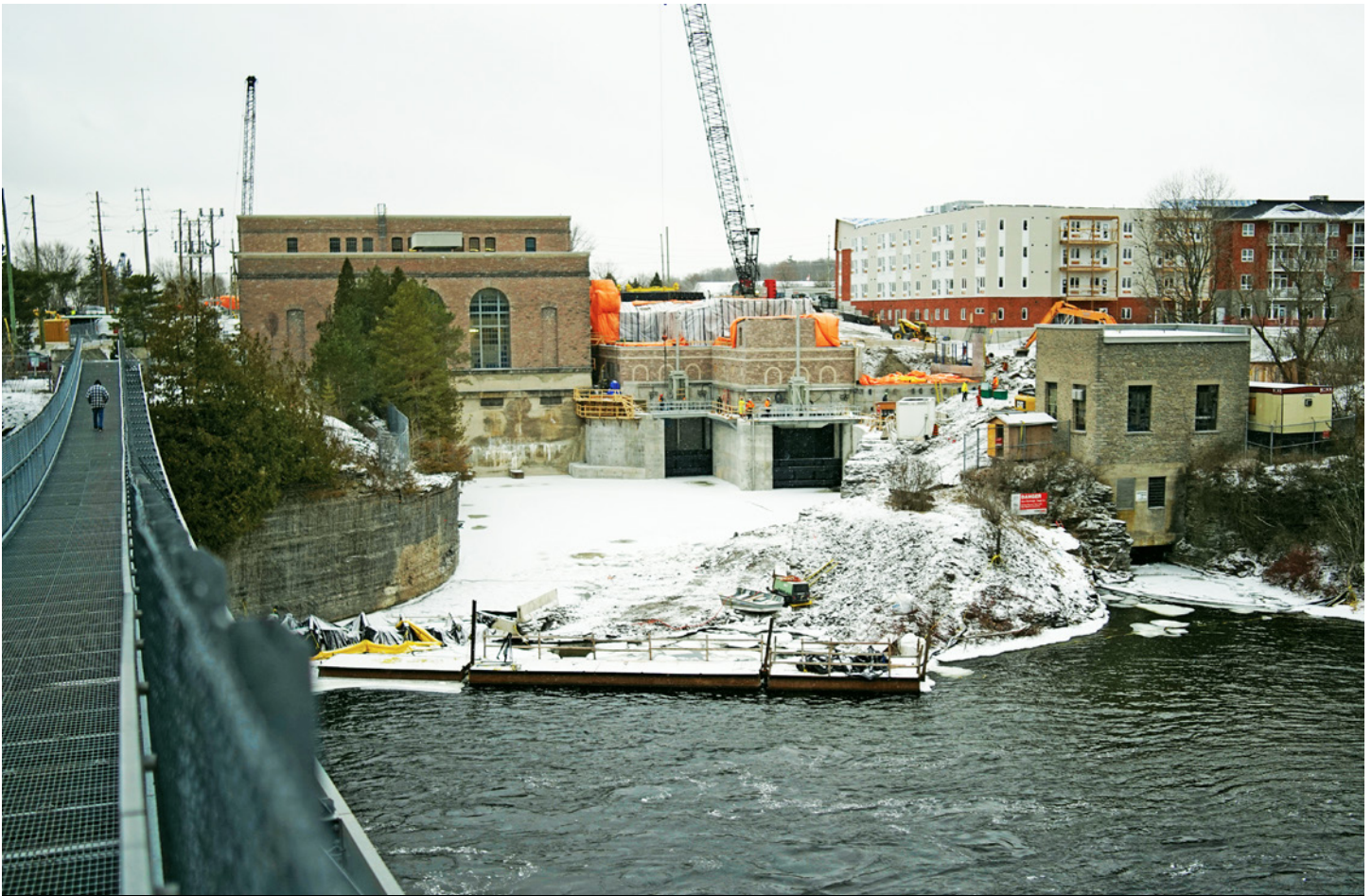
Ranney Falls Generating Station
