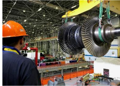
Re-installation of Lower Pressure 3 spindle
