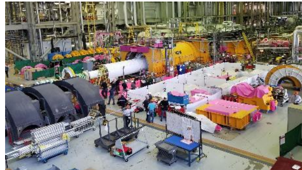
The Generator rotor being installed.
