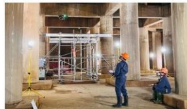
OPG employees control a drone to inspect Pickering Nuclear's vacuum building.
