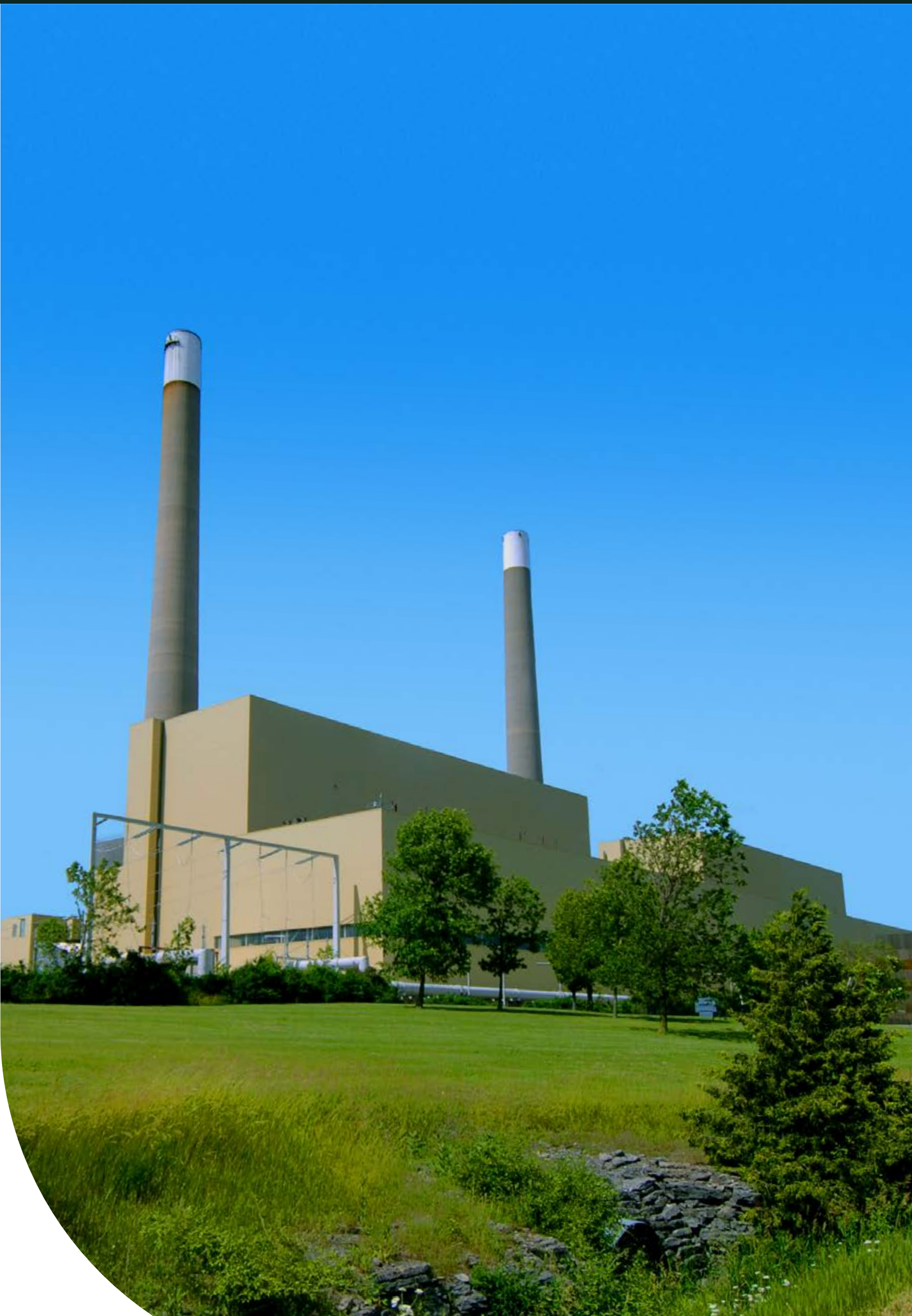
OPG's dual-fuelled Lennox Generating Station.
