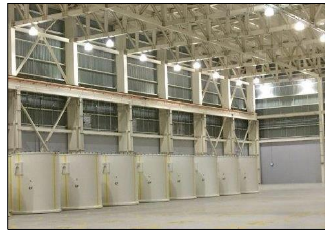
Above: Retube Waste Storage Building.
