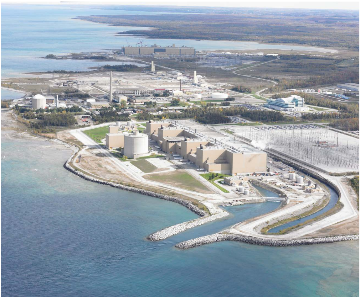
Figure 2-2: Aerial View Showing BNGS B in Foreground and BNGS A in Background
