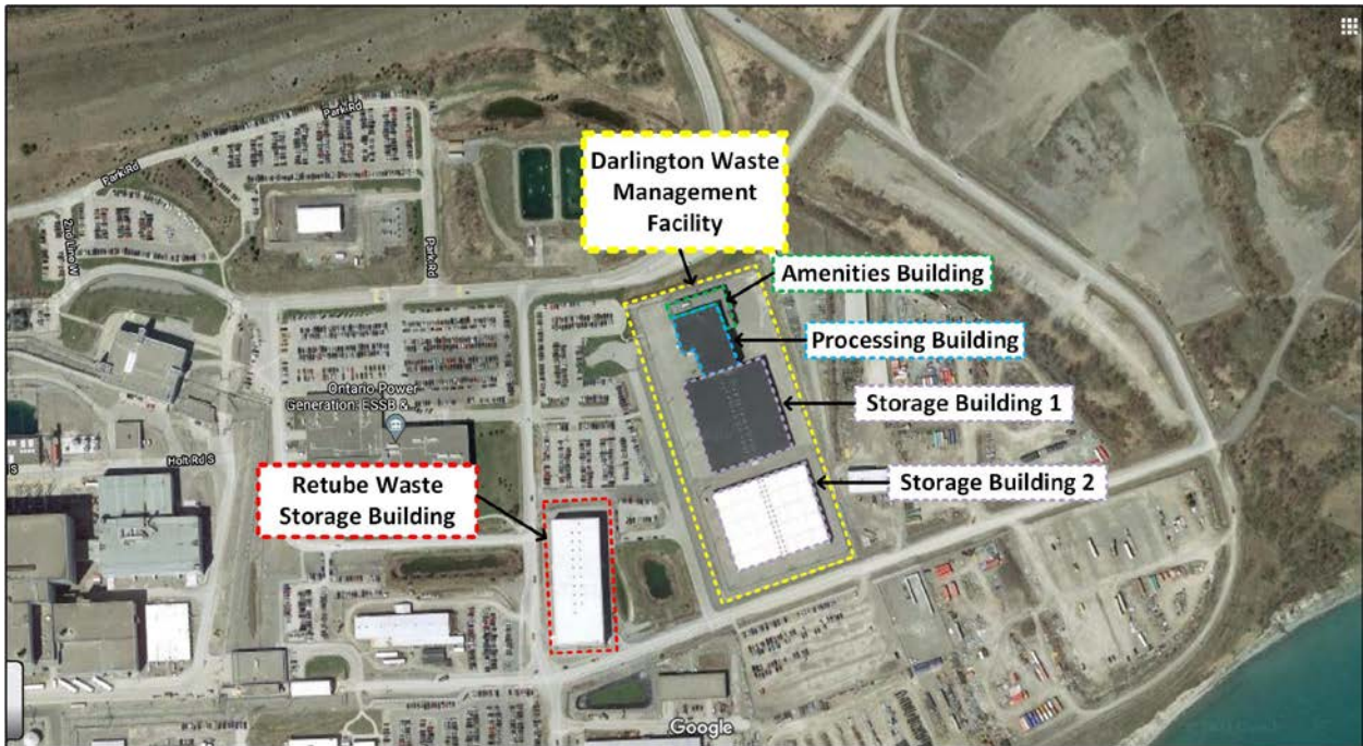
Figure 2-11: Aerial View of the Darlington Waste Management Facility
