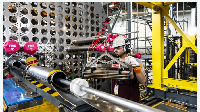
A worker practises loading one of 6,240 fuel bundles into a reactor for the Darlington Refurbishment Project at OPG's Mock-up and Training Facility. The team is scheduled to start fuelling the Unit 2 reactor this fall.
