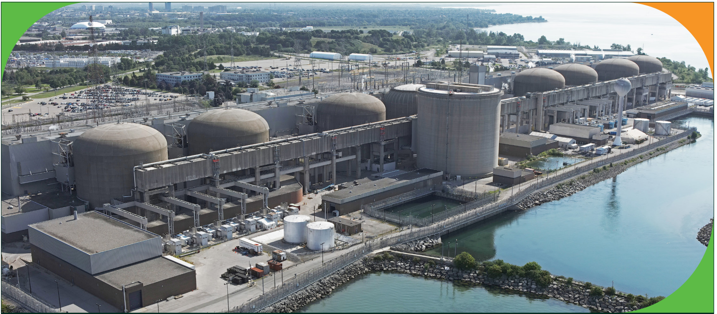
Aerial photo of Pickering Nuclear Generating Station
