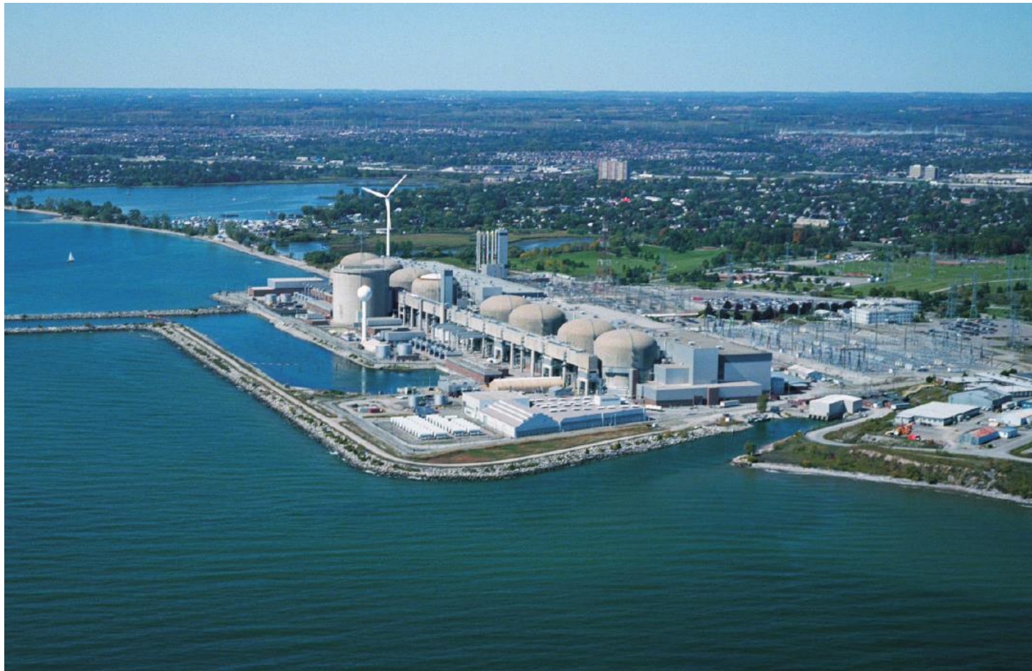
Figure 2: Aerial Photograph of Pickering Site
