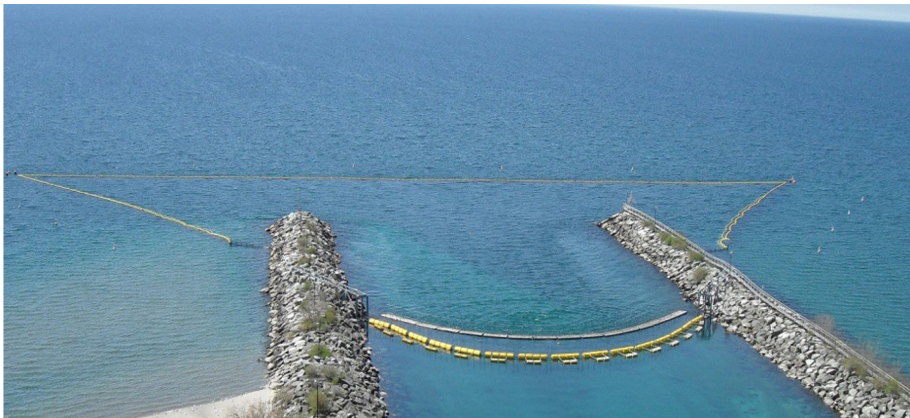
FISH DIVERSION SYSTEM
