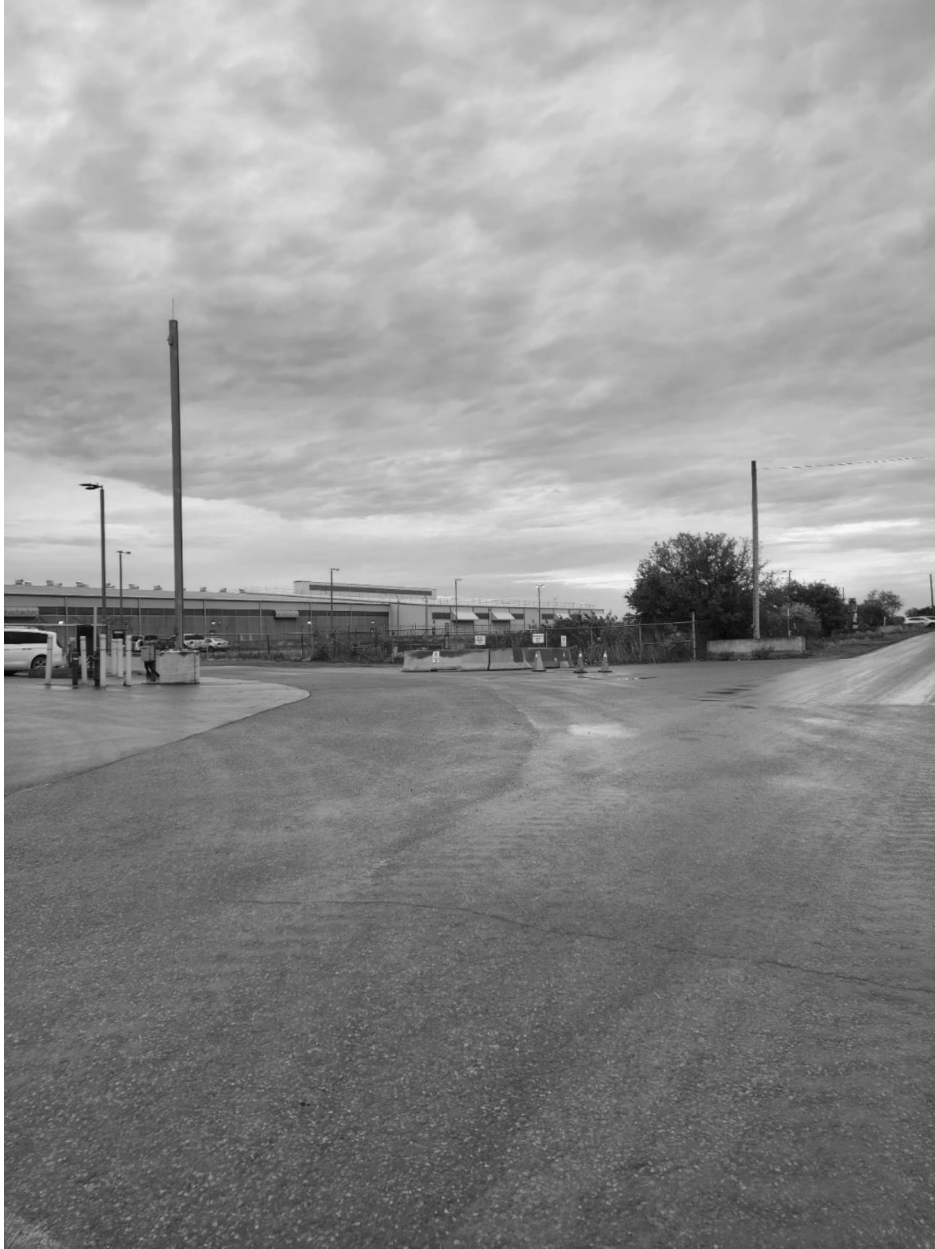
Figure C-2: Photo Taken At the Southwest Corner of East Complex Warehouse (Looking Southeast towards Entrance to PWMF Building).
