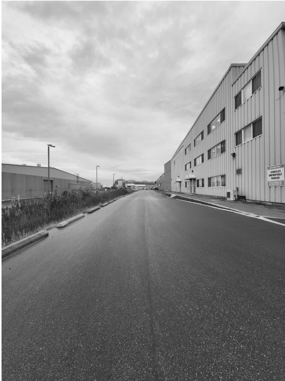
Figure C-4: Photo Taken At the Southeast Corner of East Complex Warehouse (Looking West towards PNGS).
