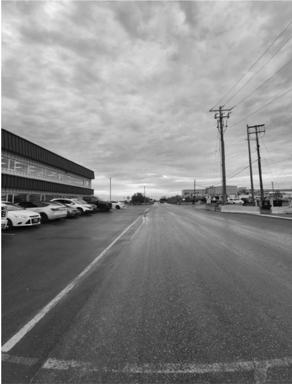
Figure C-1: Photo Taken at East Complex Warehouse Cross-Walk (Approximate 50m North of Intersection).
